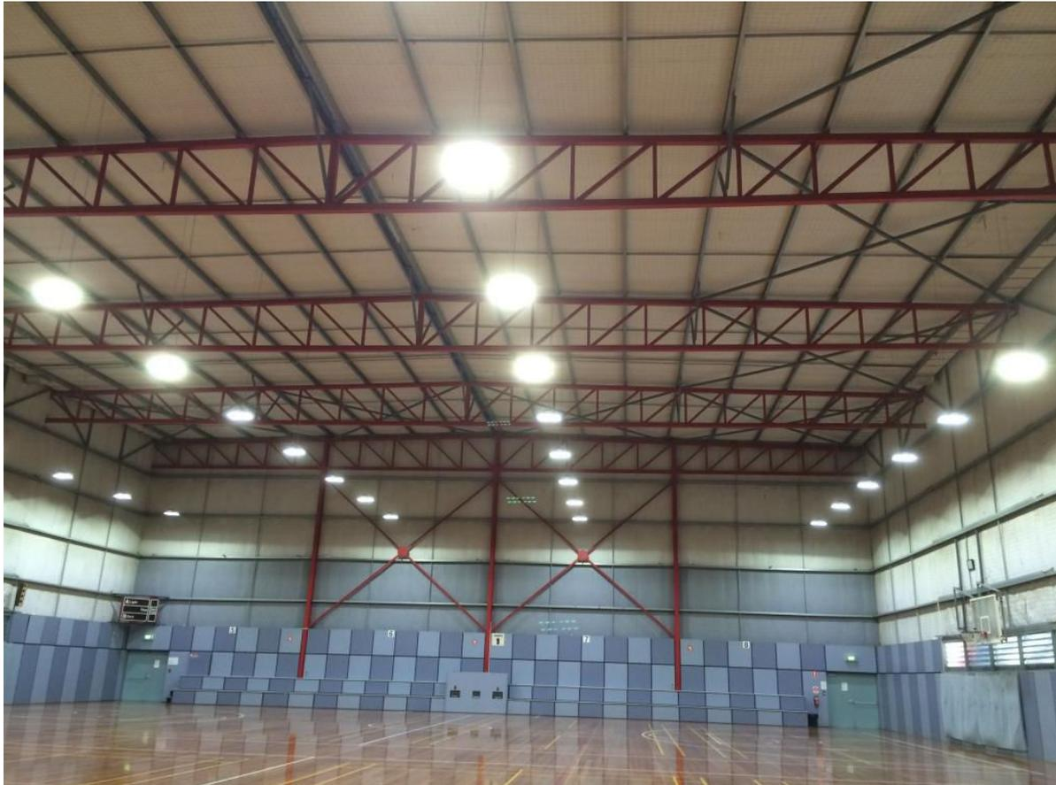
Figure 2: The image above show the contrast between the old mercury halide high bays at the front and the replacement LED lights at the rear.
