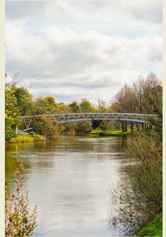
The new steel arch footbridge constructed over the Meander River.
