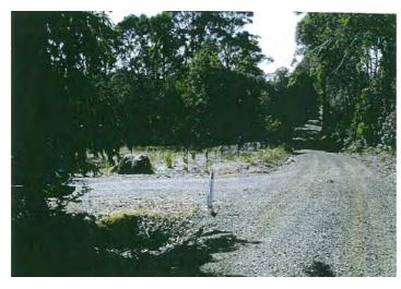
Possible turn head by culvert extension and widening driveway turn to no. 100
