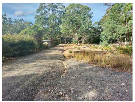
Figure 1: Washout along open drain adjacent to existing vehicle crossing within 77 Delantys Road (photo taken 22 March 2024).
