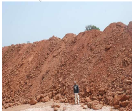
3) Absence of retaining walls, enhancing soil erosion. Girgaon
