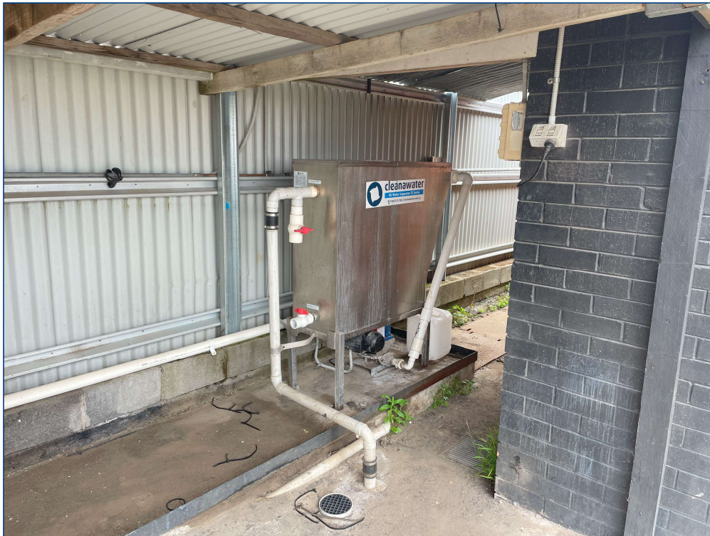
Figure 9 – Above ground oil water separator inside small bunded area
