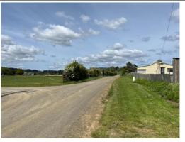
Moore Street provides a minor collector road function through the southern sections of Westbury, running in an east-west direction. It has a sealed pavement width of approximately 5 metres and a posted speed limit of 70-km/h. It carries a traffic volume of approximately 150 vehicles per day<sup>1</sup>. Jones Street connects to Moore Street at a T-junction with Moore Street having priority.
