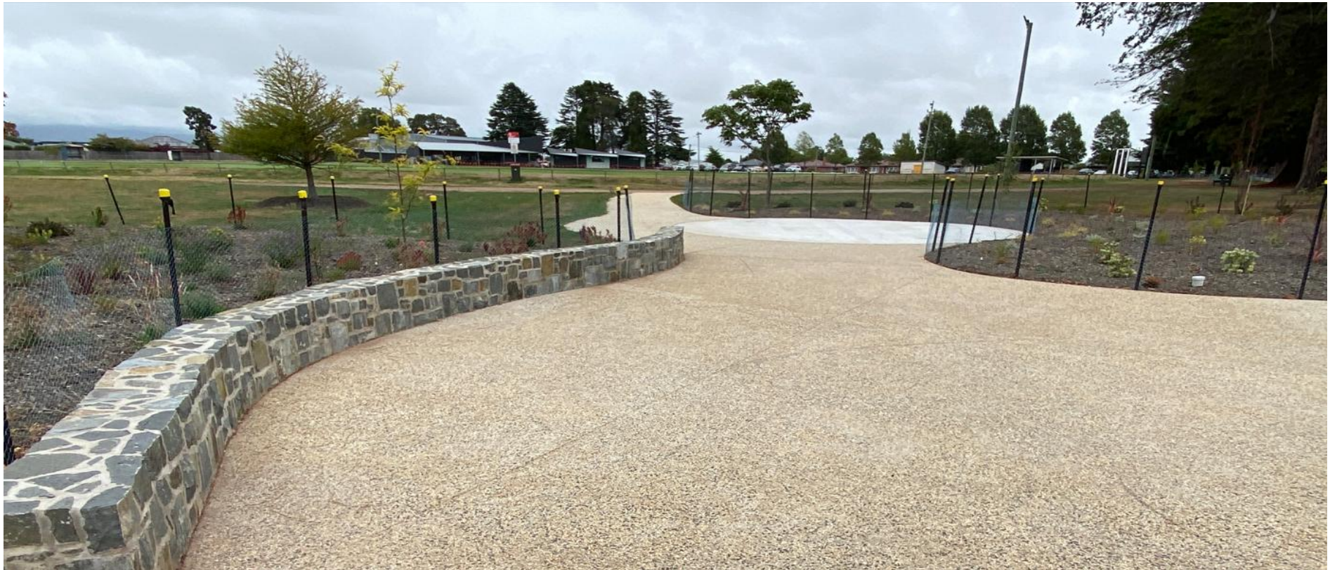
Westbury Street Scape Project - Completion of Stage 1, Franklin Street to Jones Street
