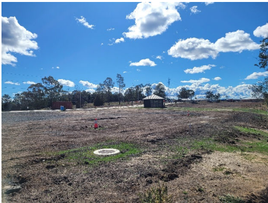
Figure 6 looking northwest over the new subdivision
