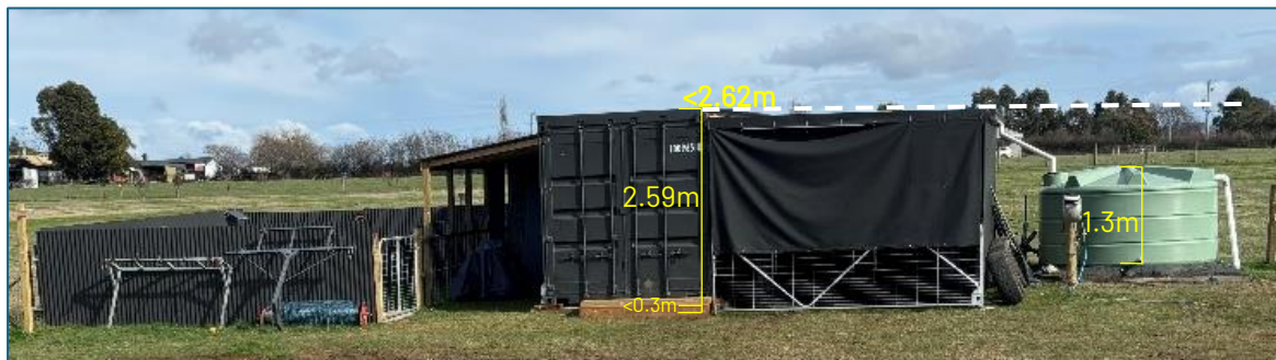
Figure 4 Detail of outbuilding structure
