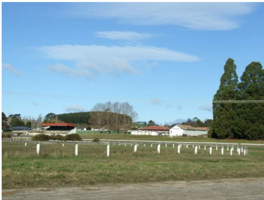
General view of the fence, track and buildings – GPA Photos 2023.
