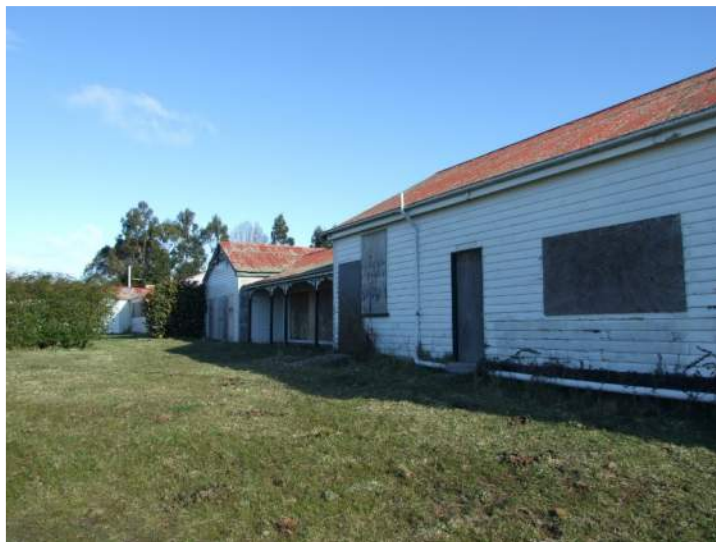
View of the buildings on south side.
