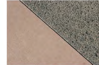
Applied colour + texture finish to existing concrete (DS)
