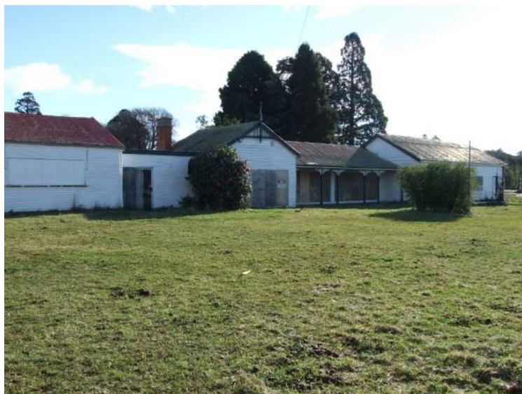
Views of the buildings on south side.
