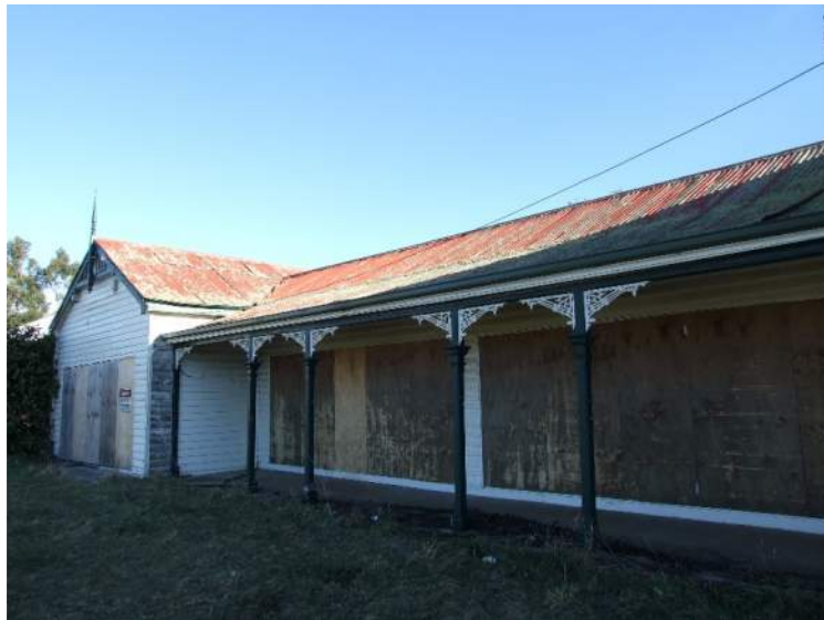
Views of the buildings on south side.
