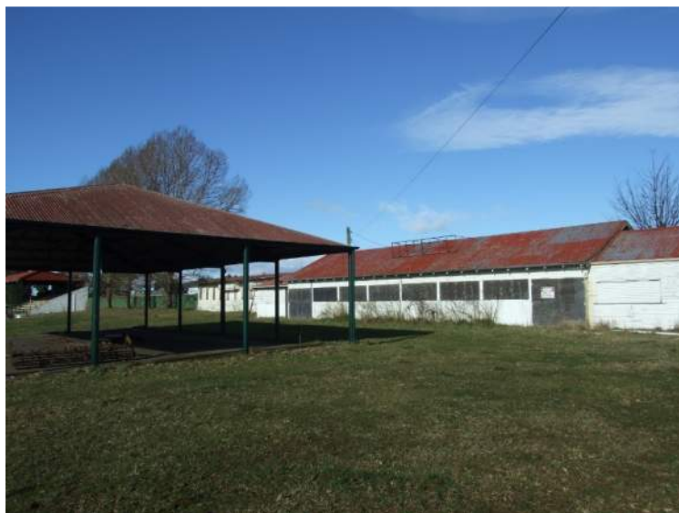
Views of the buildings on south side.
