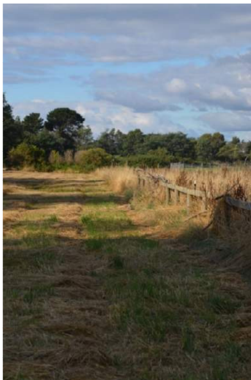
North western side fencing in poor repair – GPA Photos 2023
