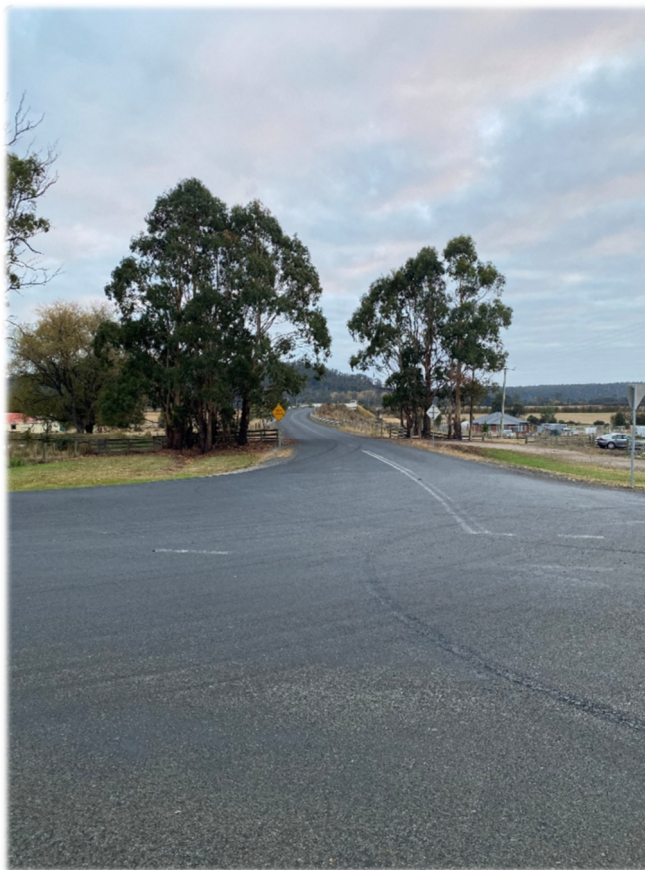
Figure 11 - Looking onto the intersection of Porters Bridge Road and Meander Valley Road
