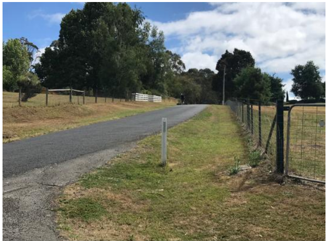
Figure 11 – Looking right along Samuel Street from Hill Street.
