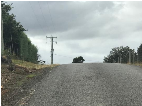
Figure 15 – Hill Street Western approach to Lot 1.
