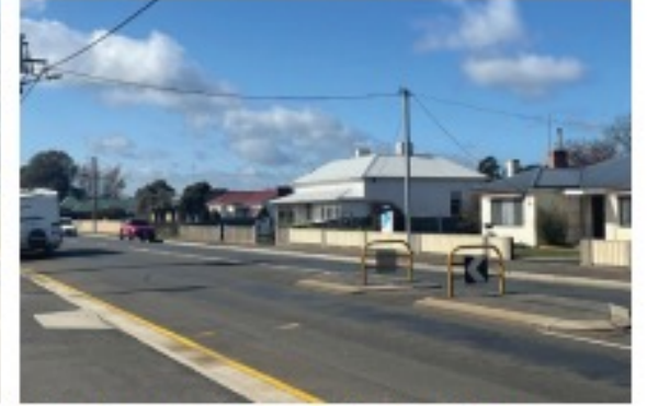
Tired crossing to IGA. Lacking visual contrast for wayfinding
