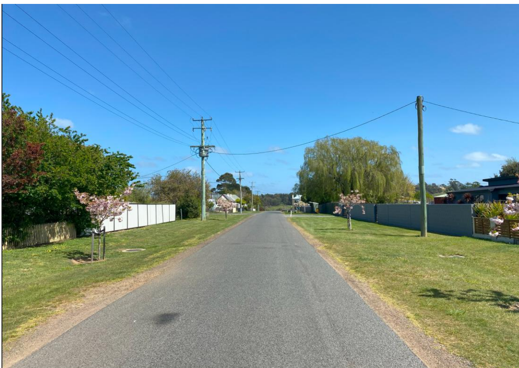
Figure 6: Liffey Street, another example of a grassed swales, narrow carriage way creating a village character (Source: David Cundall)
