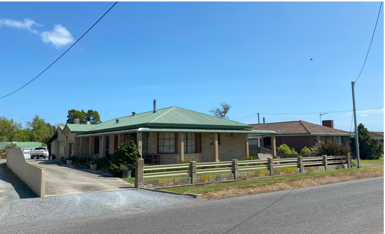
Figure 11: Dwelling built in 20 th Century using sandstone, glazing bars on windows, prominent window sills, bull nose veranda etc to create a heritage character (Source: David Cundall)
