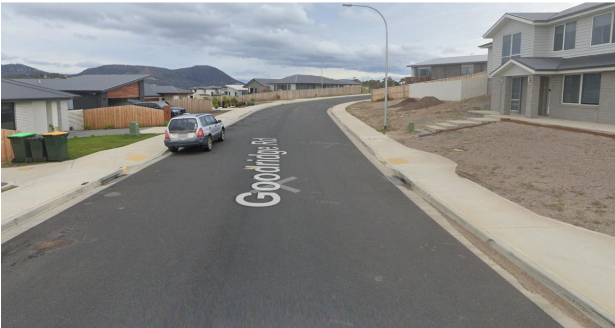
Figure 13: A recent subdivision in Goodridge Road, Austins Ferry with kerb, gutter, footpath. This is the current standard for subdivisions in residential areas (Source: Google Streetview, accessed 14 th November 2024)
