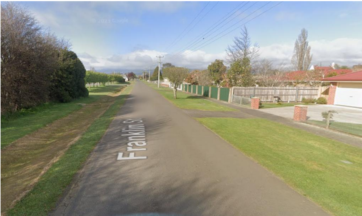
Figure 5: Grassed swales, narrow carriageway, street trees and footpath. A typical streetscape in Westbury (Source: Google Street View, September 2023)
