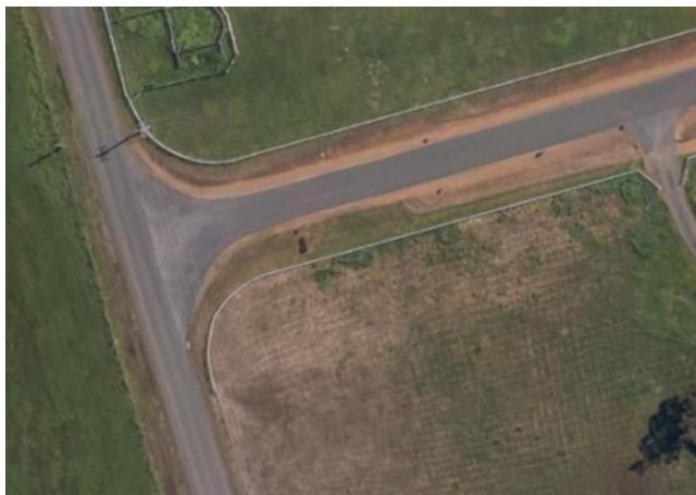
Figure 3.2.1.5 – Bishopsbourne Road / Charlies Lane junction.
