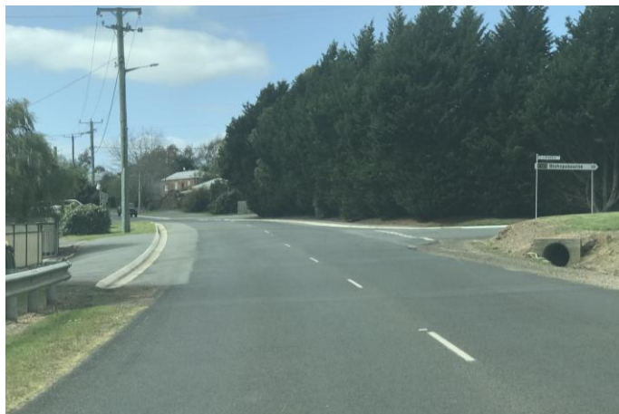
Figure 3.1.3.2 – MVR East bound lane approaching Church Street
