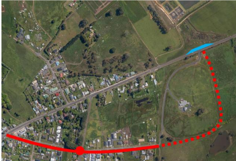
Figure 11.4.3 – Aerial view of MVR / Prop. Northern Road junction
