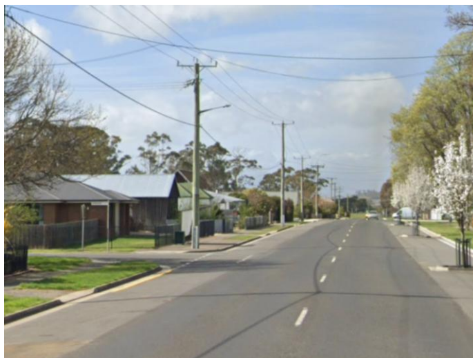
Figure 3.1.8.2 – MVR Western approach to Simmons Street
