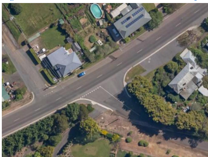
Figure 3.1.4.1 – Aerial view of MVR / South Street junction
