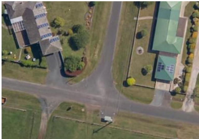
Figure 3.2.3.2 – Percy / Ashburner Street junction
