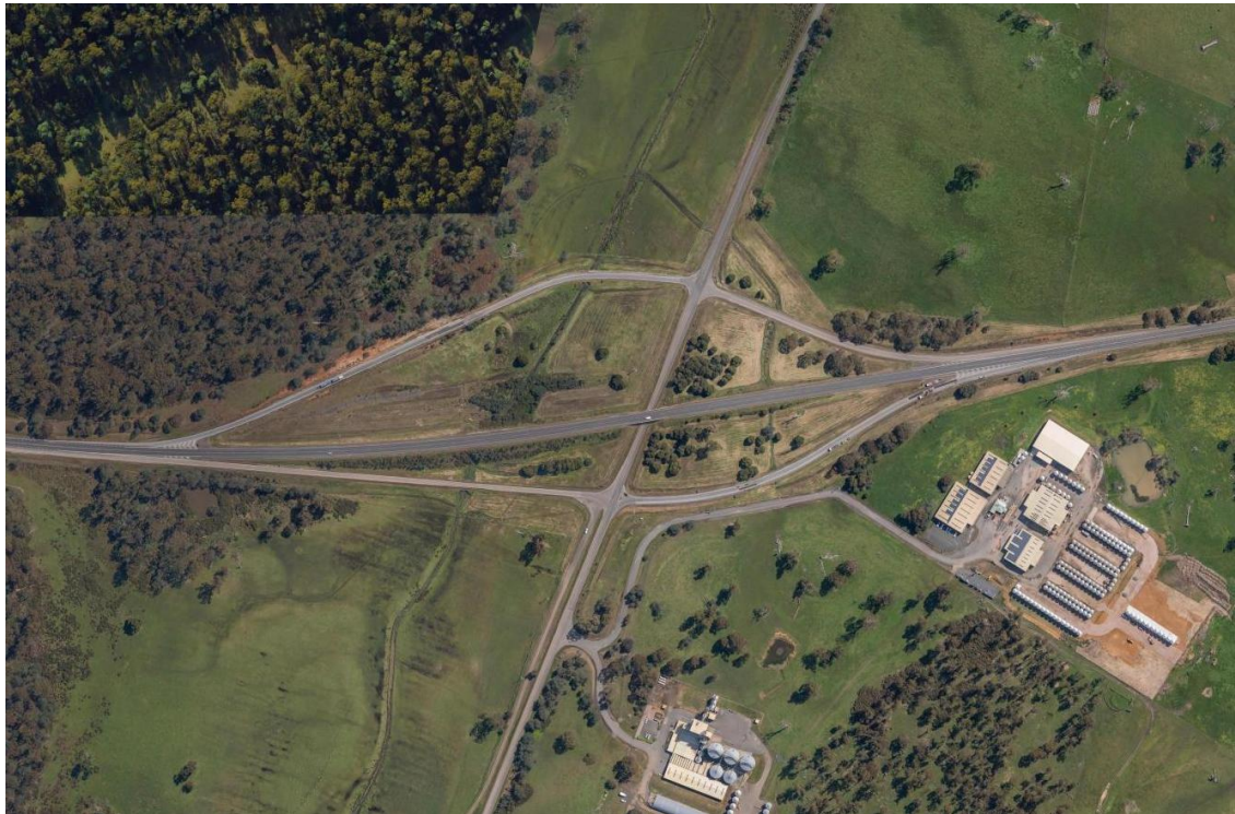
Figure 4.2 – Aerial view of Bass Hwy / Oaks Road interchange
