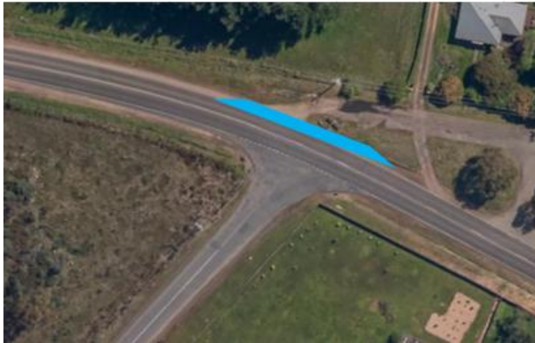
Figure 11.4.1 – Aerial view of MVR / Oaks Road junction
