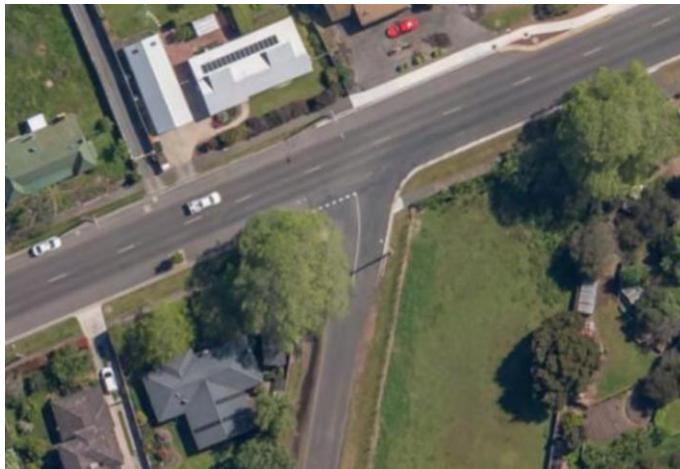
Figure 3.1.6.1 – Aerial view of MVR / East Street junction
