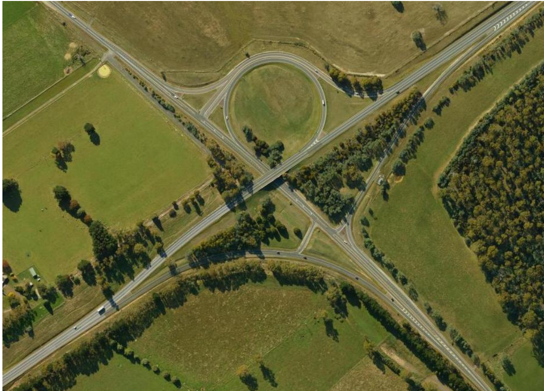
Figure 4.3 – Aerial view of Bass Hwy / Illawarra Road interchange
