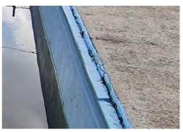
Figure 4: Cracked Hob Paver (west side)
