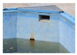
Figure 7: Skimmer & Low Level Suction Point
