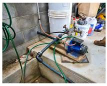
Figure 14: Make-up Water Pump
