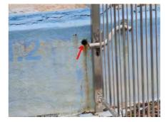
Figure 15: Pump Discharge Line into Pool
