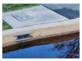
Figure 6: Outdoor Toddler Pool Concrete Surface Pitting & Leaching
