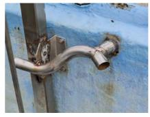
Figure 8: Filtered Water Return Inlet
