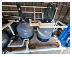
Figure 23: 25m Pool Pipework (supported on bricks)
