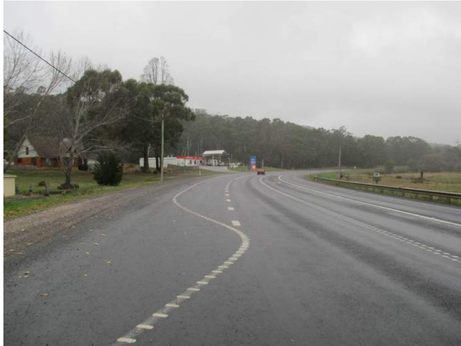
Photograph 4.1: View to south along Bass Highway with service station site ahead on left
