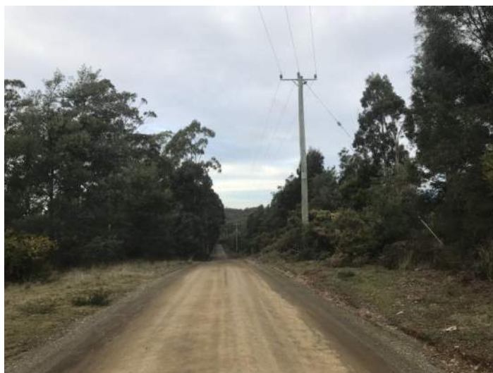
Figure19 – Looking south along Wadleys Road with power poles on the western side.
