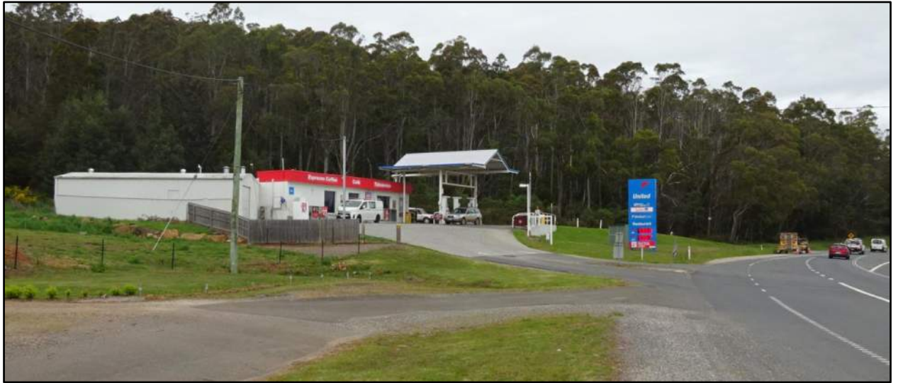
Photo 1: Subject site, showing the existing service station, viewed from the north.
