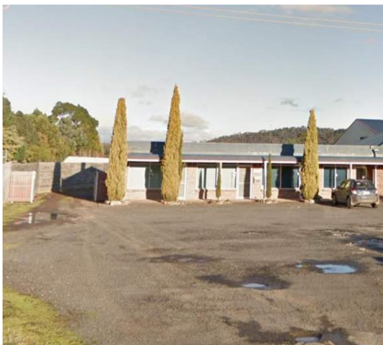
Photos of the already established retail shopfronts at 8 Neptune Drive, Blackstone Heights.
