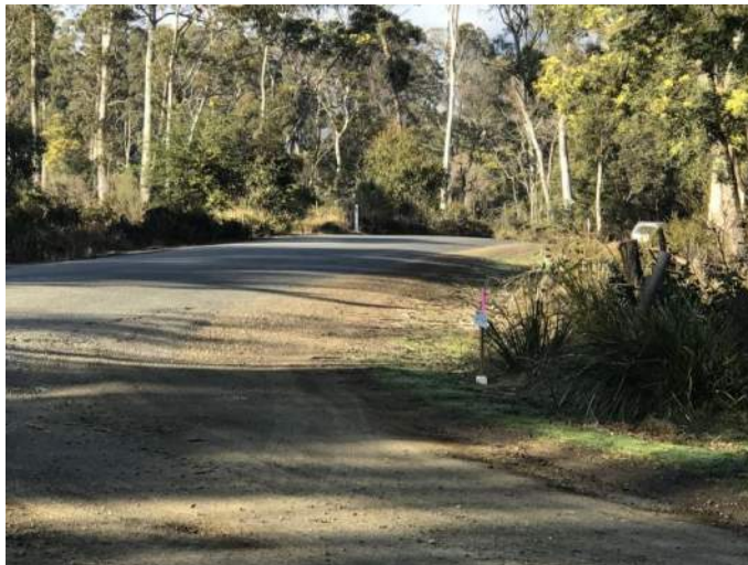
Figure 7 – Looking west along River Road from Wadleys Road northern approach
